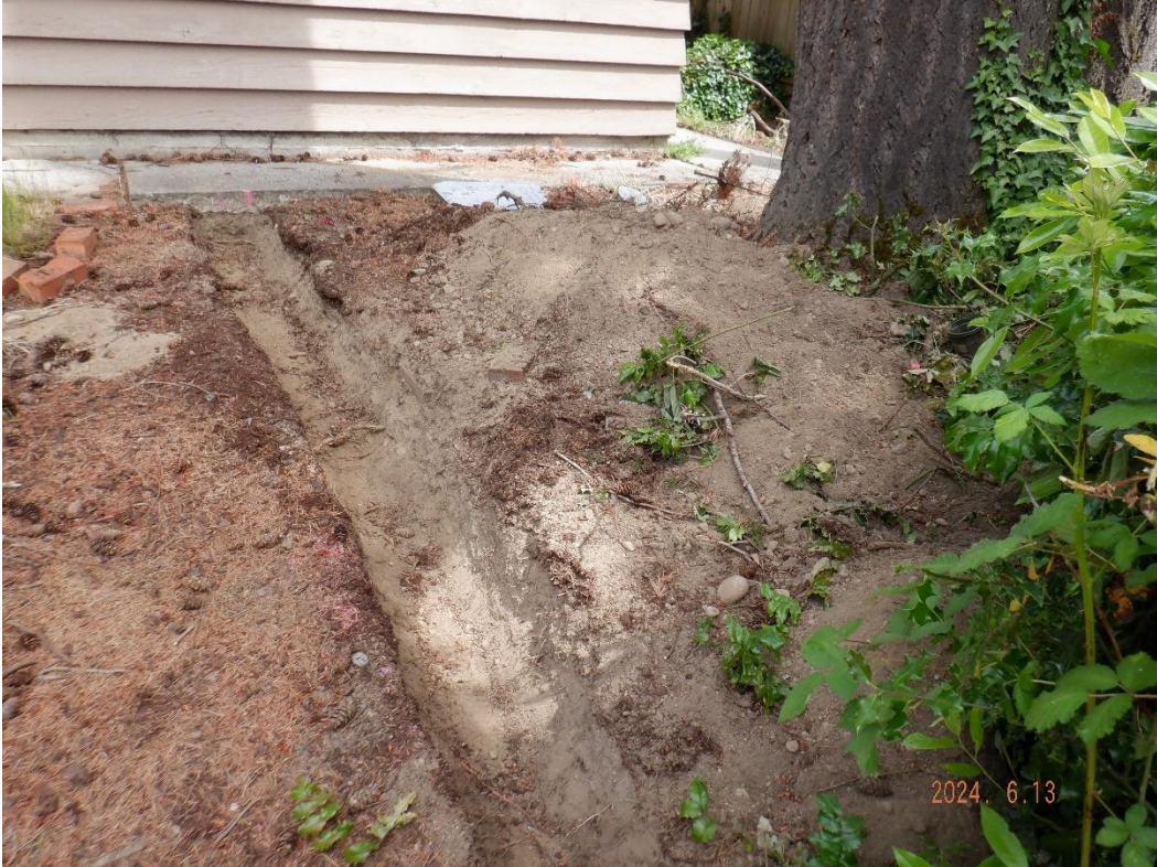
Hand-excavated trench 5-feet from trunk face of Tree #7
