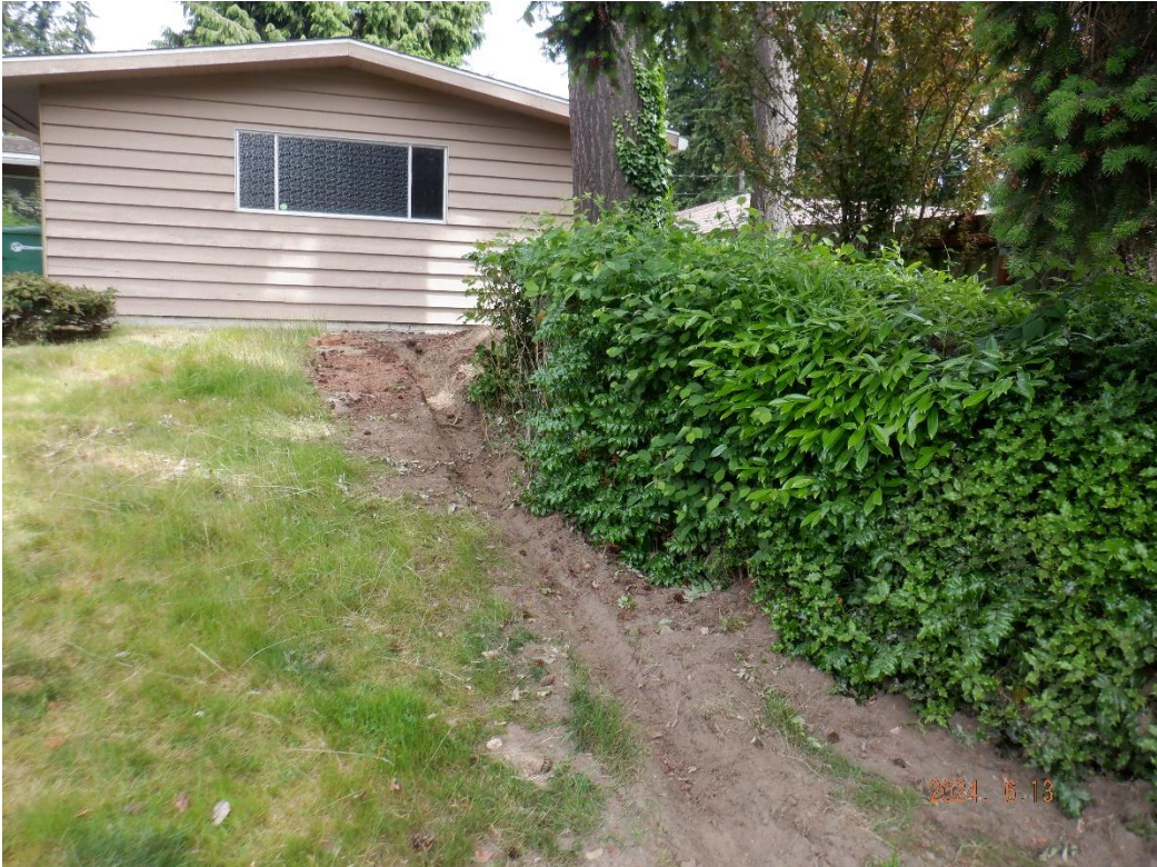
Hand-excavated trench at edge of proposed new driveway
